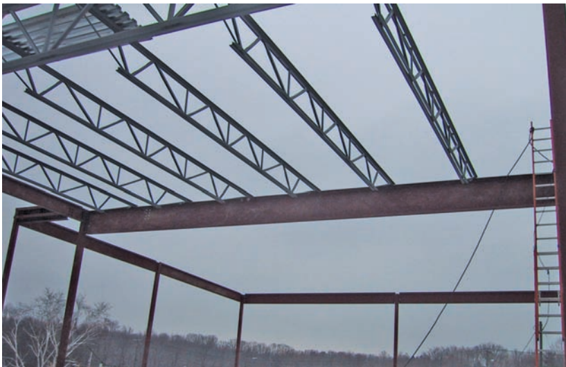
Photo 9.2 In this roof structure, each of the open-web joists applies a concentrated load to the beam that supports it.
