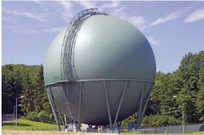
Photo 7.2 Spherical pressure vessel.
