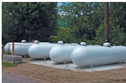
Photo 7.3 Cylindrical pressure vessels for liquid propane.
